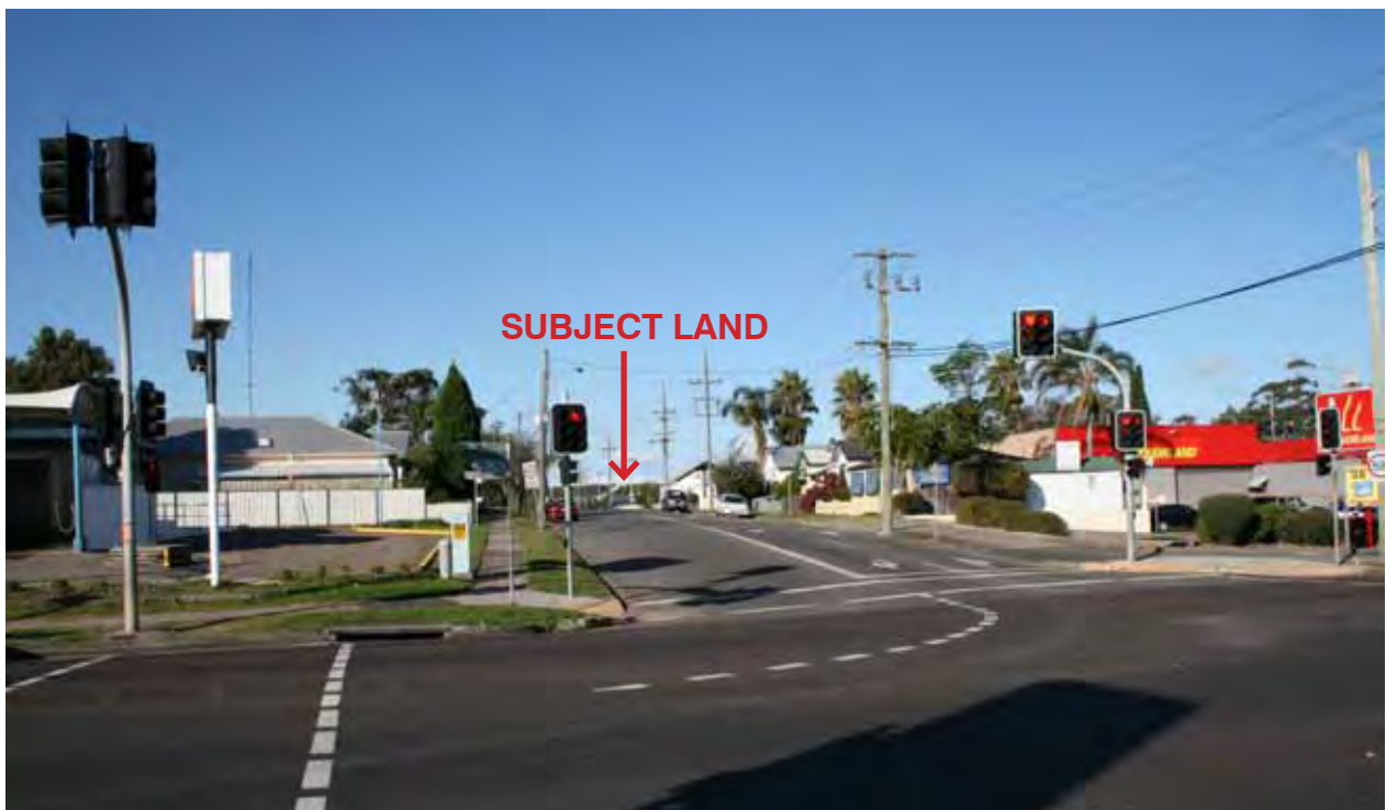
Figure X. Looking towards the proposed development from the Pacific Highway
