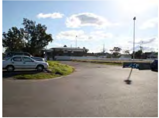
Photo X. Bowling greens as viewed from the rear car park
